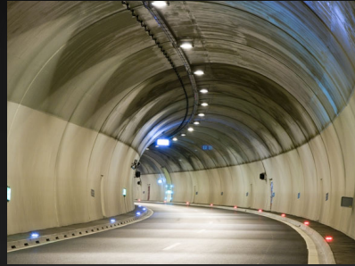
Highways and Road Tunnels
