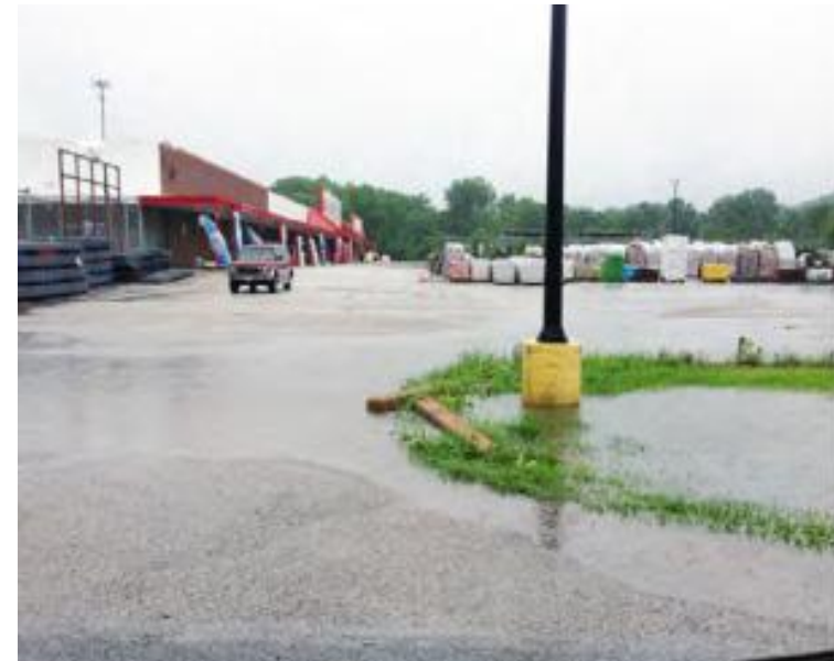
Figure 22: Examples of Stormwater Issues at Rural King (9525 Collinsville Road)
