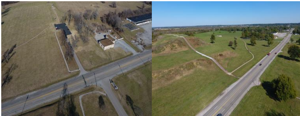
Figure 19: Existing Conditions at Cahokia Mounds
