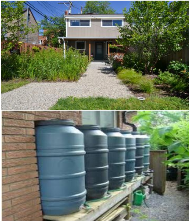
Figure 26: Examples of Private Stormwater Management
