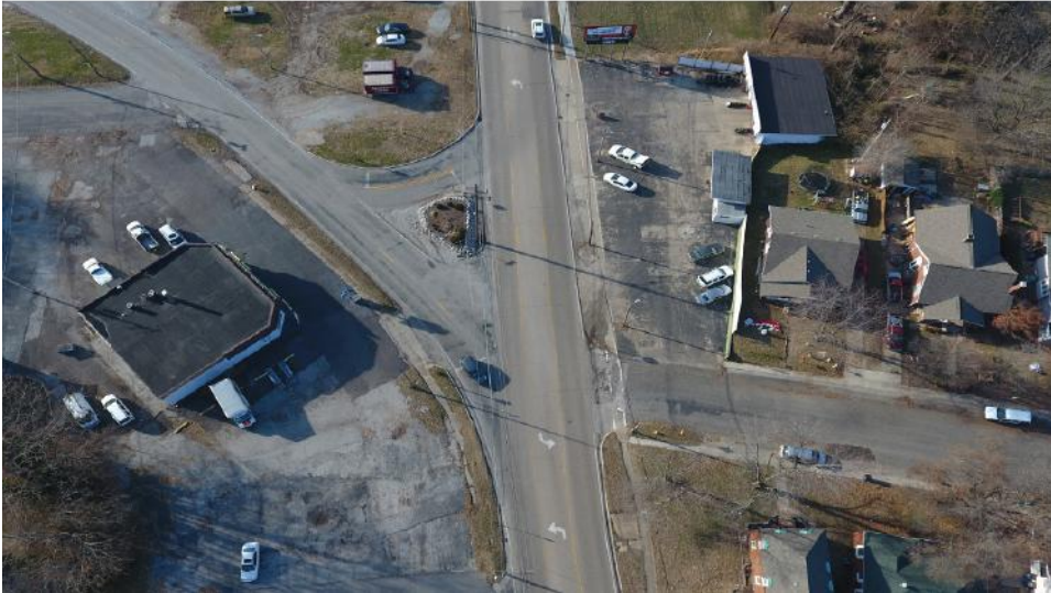
Figure 14: Collinsville Road between Highway 157 and Interstate 255
