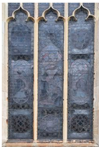
Another south aisle window showing multiple sites of bowing in the window.
