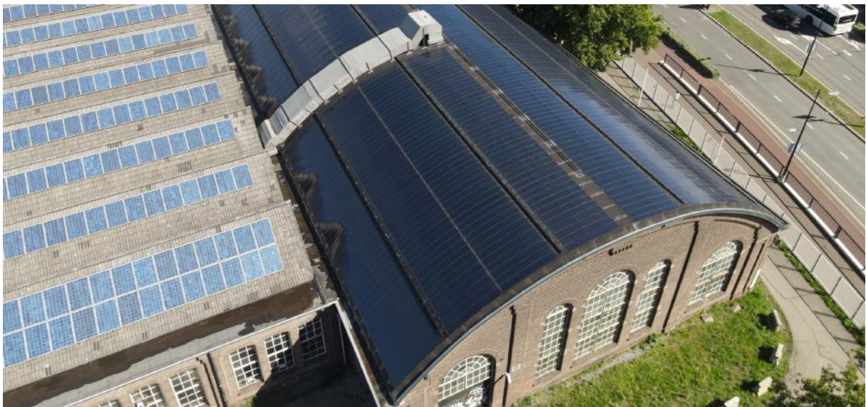
Flexibele panelen Koepelhal Tilburg
