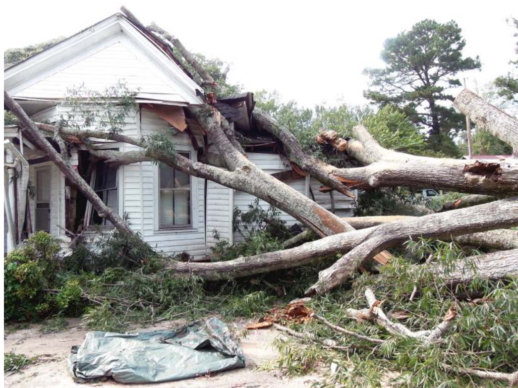
This tree damaged a house on Orange Street in Abbeville last week. Torrential rains contributed to the accident, in which no one was hurt. (Staff photo by Henry E. Green)
