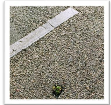
Concrete #VPCMc4 High Voltage
