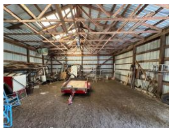
POLE BARN: 32' x 40' x 12' | Built 1979
