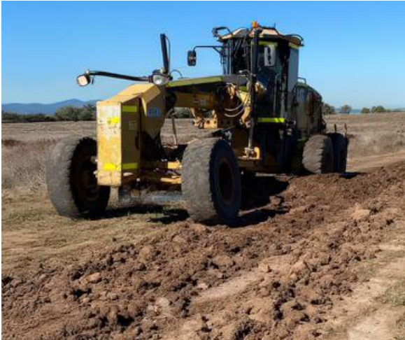
Machinery operators forming horseshoe-shaped banks.
