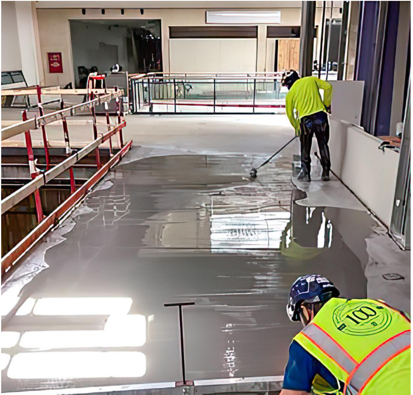
Every surface receiving tile, stone, or terrazzo was surveyed for substrate suitability. Many required correction—especially in repurposed shopping mall areas with damaged concrete.
