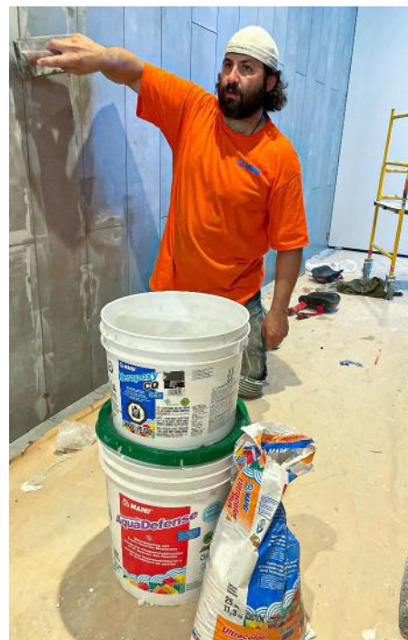
An installer applies MAPEI's Ultracolor Plus FA grout, selected for its fast-setting, stain-resistant formula that delivers a durable, color-consistent, and low-maintenance finish throughout The Spiral. Photo: Bjarke Ingels Group (BIG)
