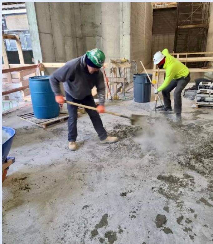
Crew members install 4 to 1 Mud Bed Mix enhanced with Planicrete AC, creating a stable, level foundation with superior bond strength and long-term durability for The Spiral's flooring installations. Photo: Bjarke Ingels Group (BIG)
