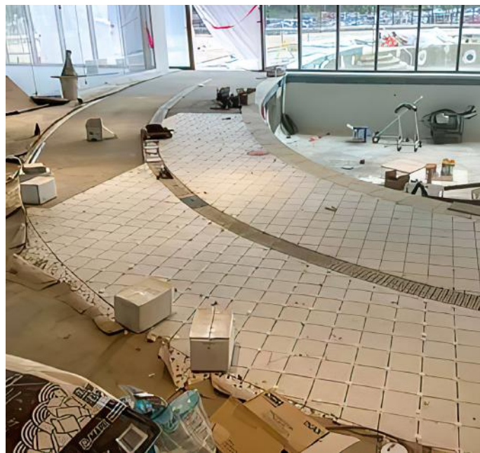
Crews tiled the pool deck in just five days after the concrete pour, using a rapid-curing epoxy vapor barrier.
