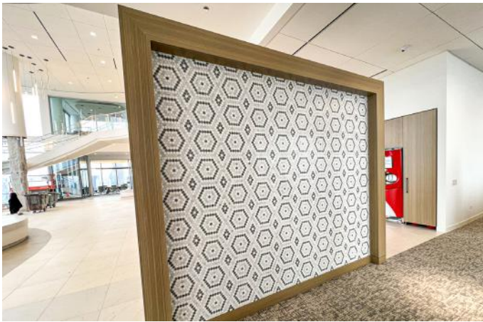
The cafe includes a full-height 1" hexagon mosaic backsplash, while 30' away, the atrium showcases a two-sided feature wall clad in full-height 1"x1" hexagon marble mosaic.
