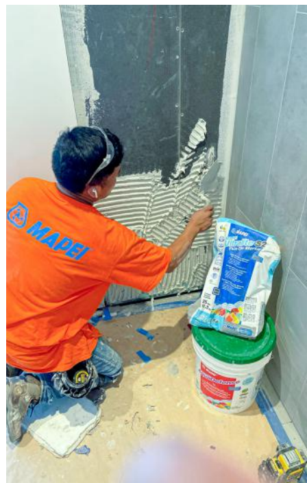
An installer applies MAPEI Ultralite S2 lightweight mortar, delivering exceptional adhesion and flexibility for the large-format tiles featured throughout The Spiral. Photo: Bjarke Ingels Group (BIG)
