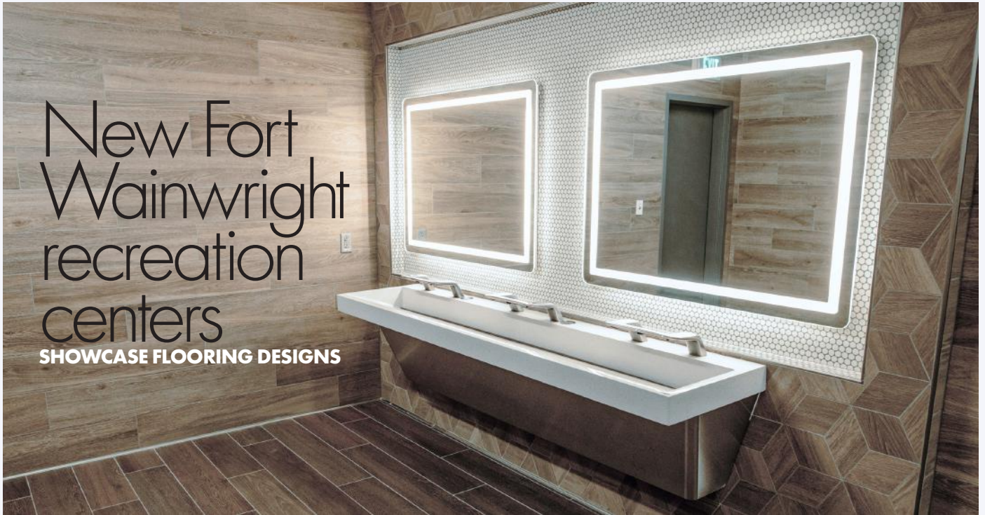
Penny tile accents, wood-look 3D illusion tile cubes and shadow boxes were used around the sinks and mirrors. TEC® 3N1® Performance Mortar was chosen for its outstanding vertical grab.
