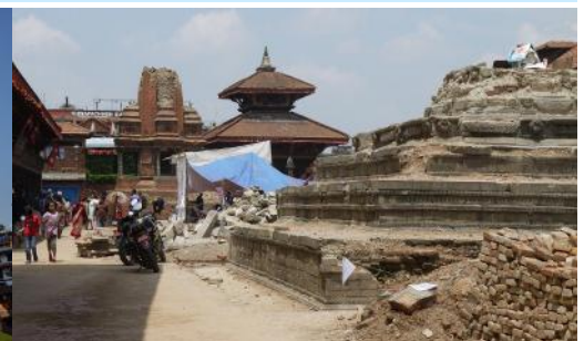
Massive destruction in Bhaktapur Darbar square
