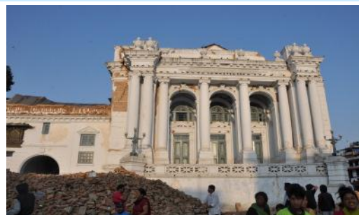
Scene of destruction in Basantapur Darbar square.
