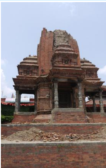
One of the destroyed temple in Bhaktapur Darbar square.
