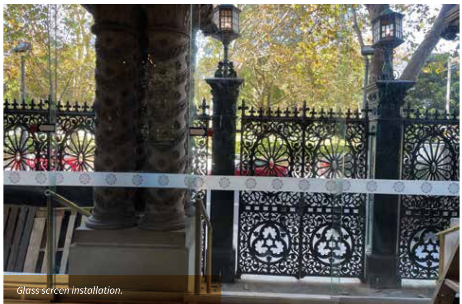
Disability Lift installation complete.
