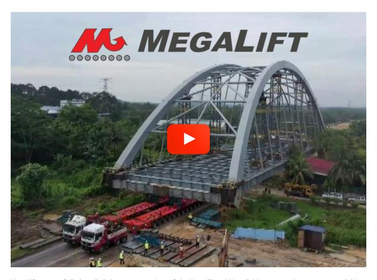
Megalift successfully handled the transportation of the Kota Tinggi New Bridge, a massive structure weighing 1,700 tons, using 168-axle multi-axle Goldhofer trailers and 4 SPT power packs.
