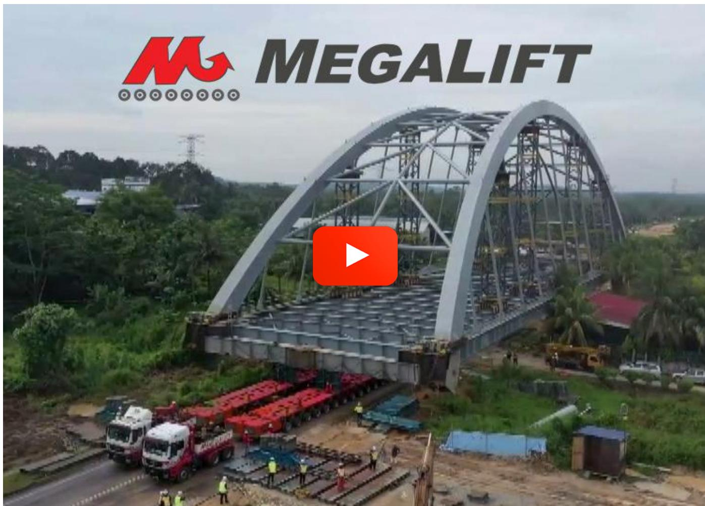
Megalift successfully handled the transportation of the Kota Tinggi New Bridge, a massive structure weighing 1,700 tons, using 168-axle multi-axle Goldhofer trailers and 4 SPT power packs.
