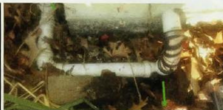
line going to pool (one foot below ground)
