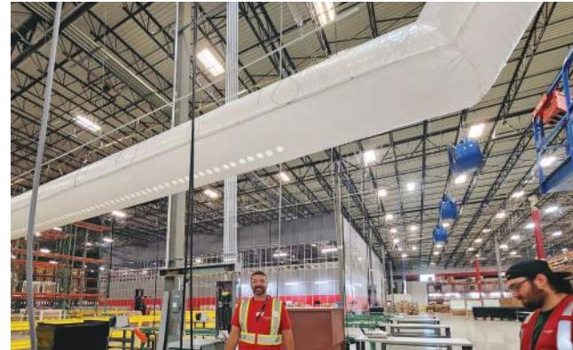
The Patterson Power Tube is a fabric air duct system custom-designed to efficiently control airflow distribution over large areas by directing air through a custom-vented tube powered by one of Patterson's High-Velocity Fans. One fan can send airflow across multiple workstations or down an assembly line to several workers at floor level.
