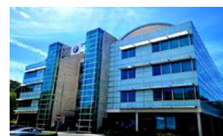
BMW Group Headquarters in Farnborough
