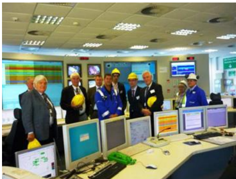
The Control Room at Didcot B
