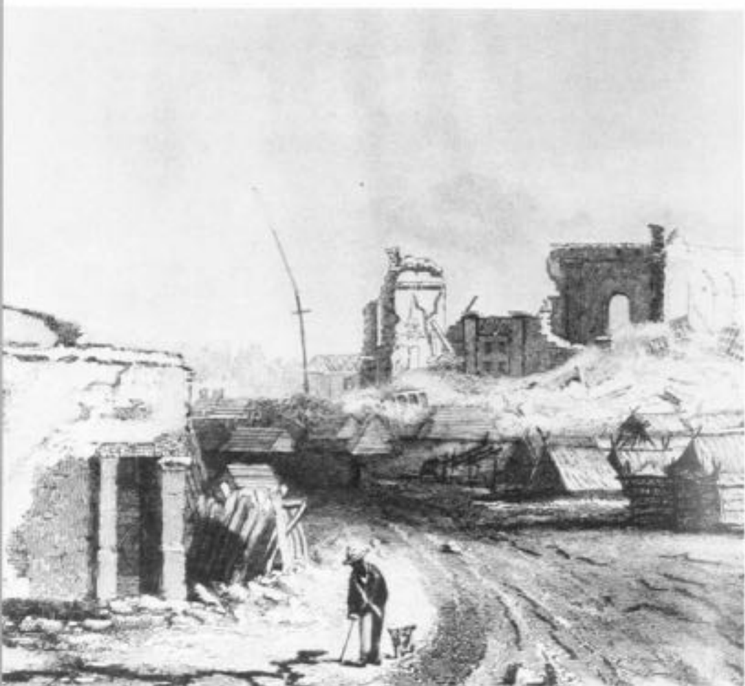
Earthquake damage in Concepción, Chile, February 1835
