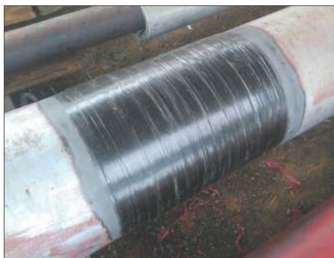
Image 6: A Belzona SuperWrap II application before being overcoated with Belzona 5811 (Immersion Grade) for extra protection.
