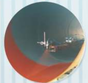
Internal pipe coating
