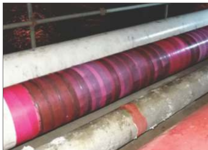
Image 4: The pipe repair before the removal of the release film.
