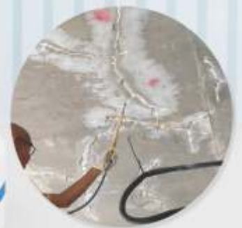
Injection Grouting
