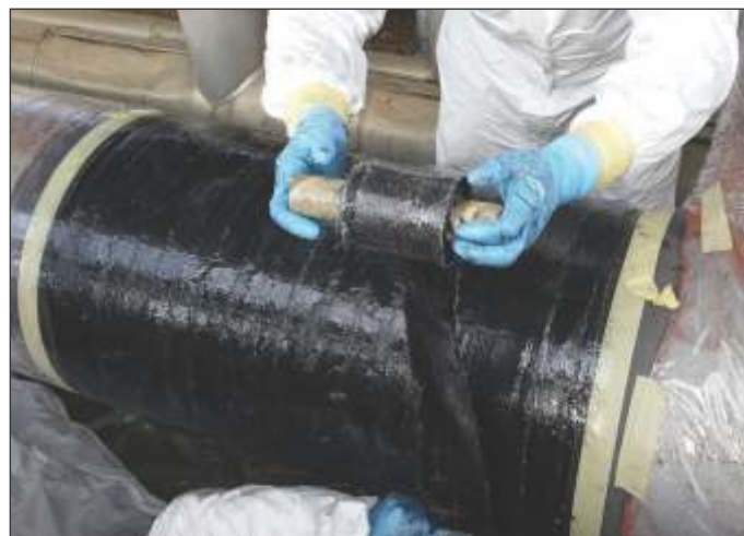
Image 5: Belzona SuperWrap II being applied.
