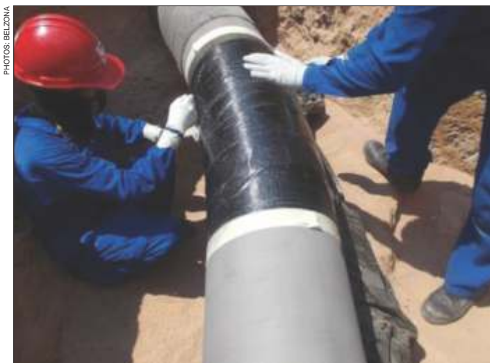
Image 1: In-field application of Belzona SuperWrap II on a corroded pipeline.
