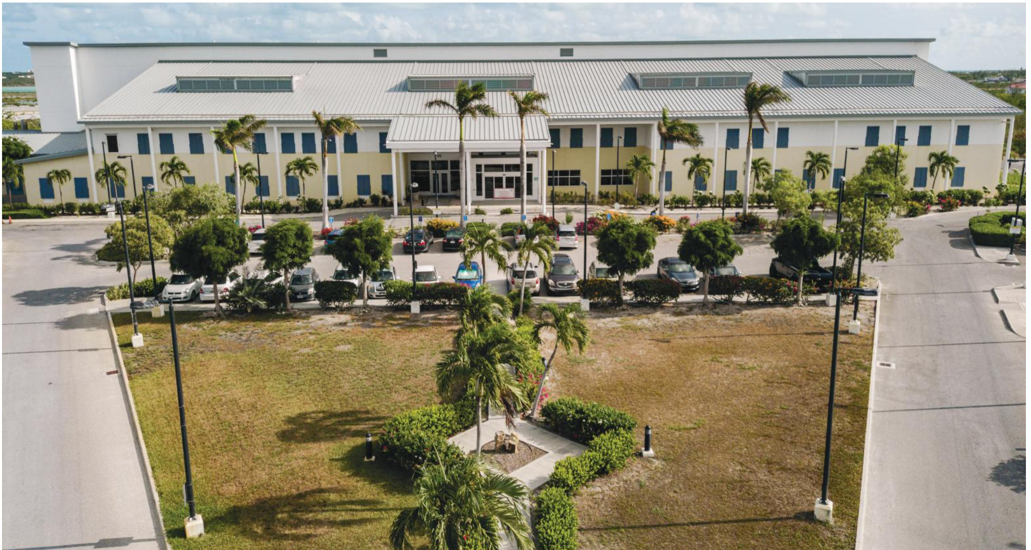
The Cheshire Hall Medical Centre in Providenciales
