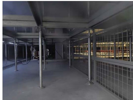
An example of mesh infill between the building floor and the computer floor.
