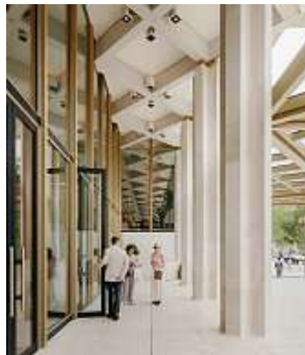
Above Grand, 4.5m-high Portland stone-clad concrete columns support the diagrid at its perimeter. Double-height aluminium double-glazed units vastly improve the facade's thermal efficiency.
