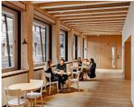
Above and top Following cradle-to-cradle values, all components were catalogued for reuse, with metal connections avoided in timber joinery.
