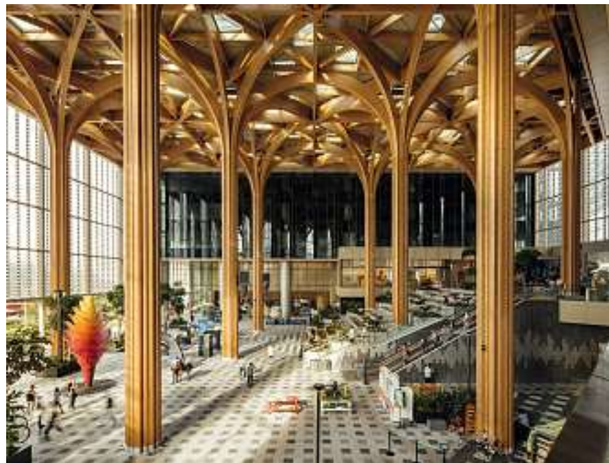
Below The Canopy at Geneo, a 3,000m 2 event plaza with a glulam arched roof structure at the Singapore Science Park.
