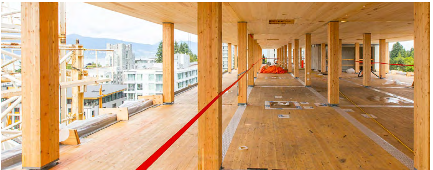
Point-supported CLT floors on glue-laminated timber columns
