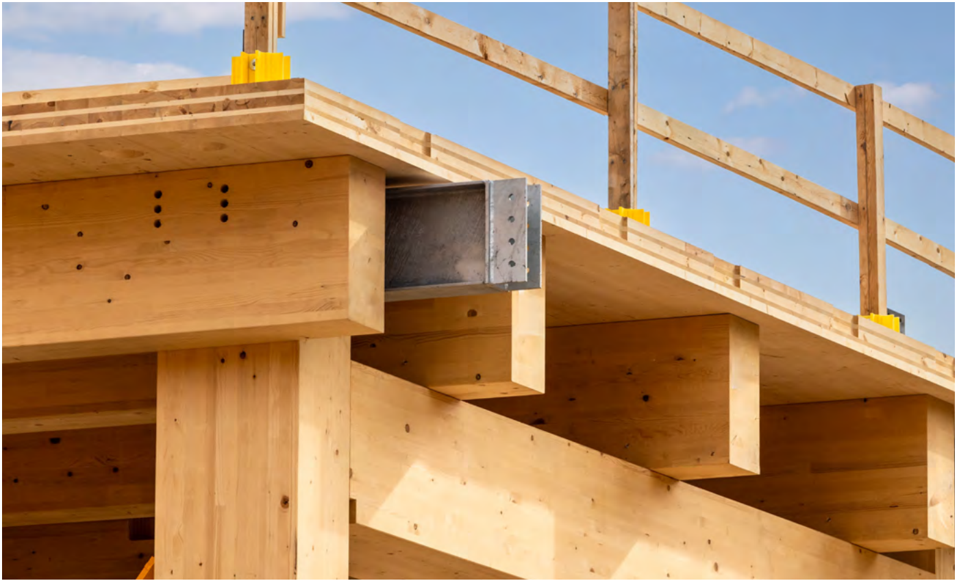
Cross-laminated timber (CLT) floor panel on glue laminated beams.
