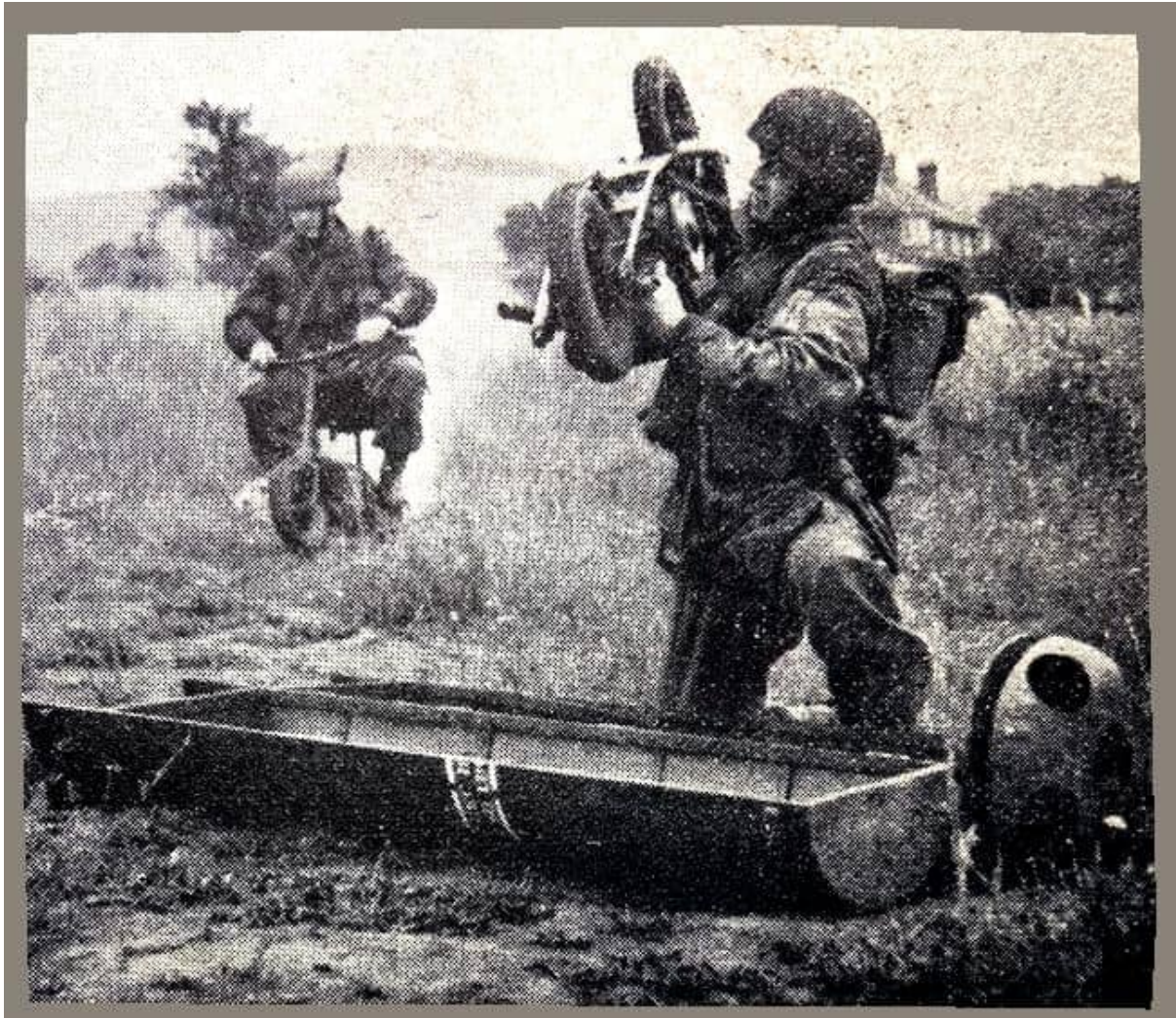
“CONTAINER JOBS.—A British official picture of one of the Excelsior ‘Wellbikes’ being removed from its parachute container. These scooter-like machines which have been issued to parachute brigades weigh under 80lb and, like autocycles, whose 98cc Villiers engine unit they possess, have a single gear.”
