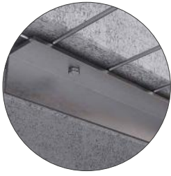
steel angle bracket 30 x 30 x 3 mm
