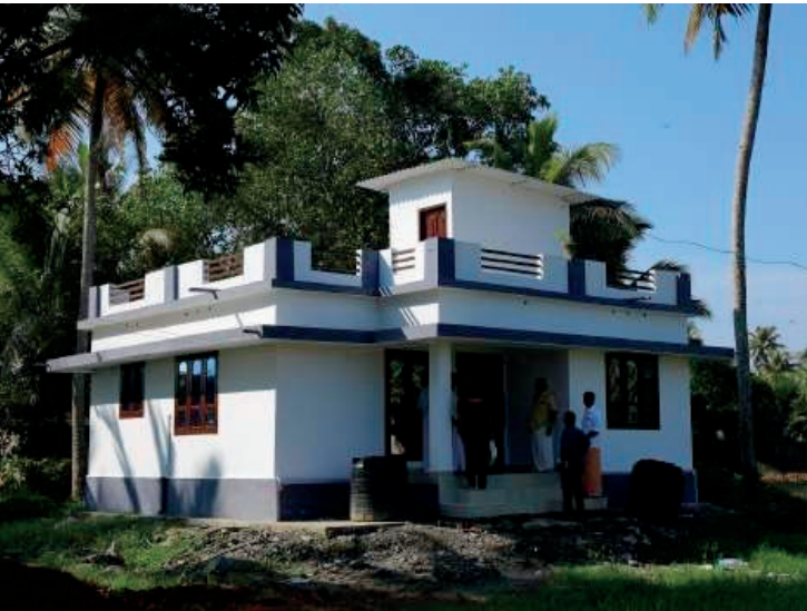
House constructed for the beneficiaries as part of the rehabilitation efforts.
