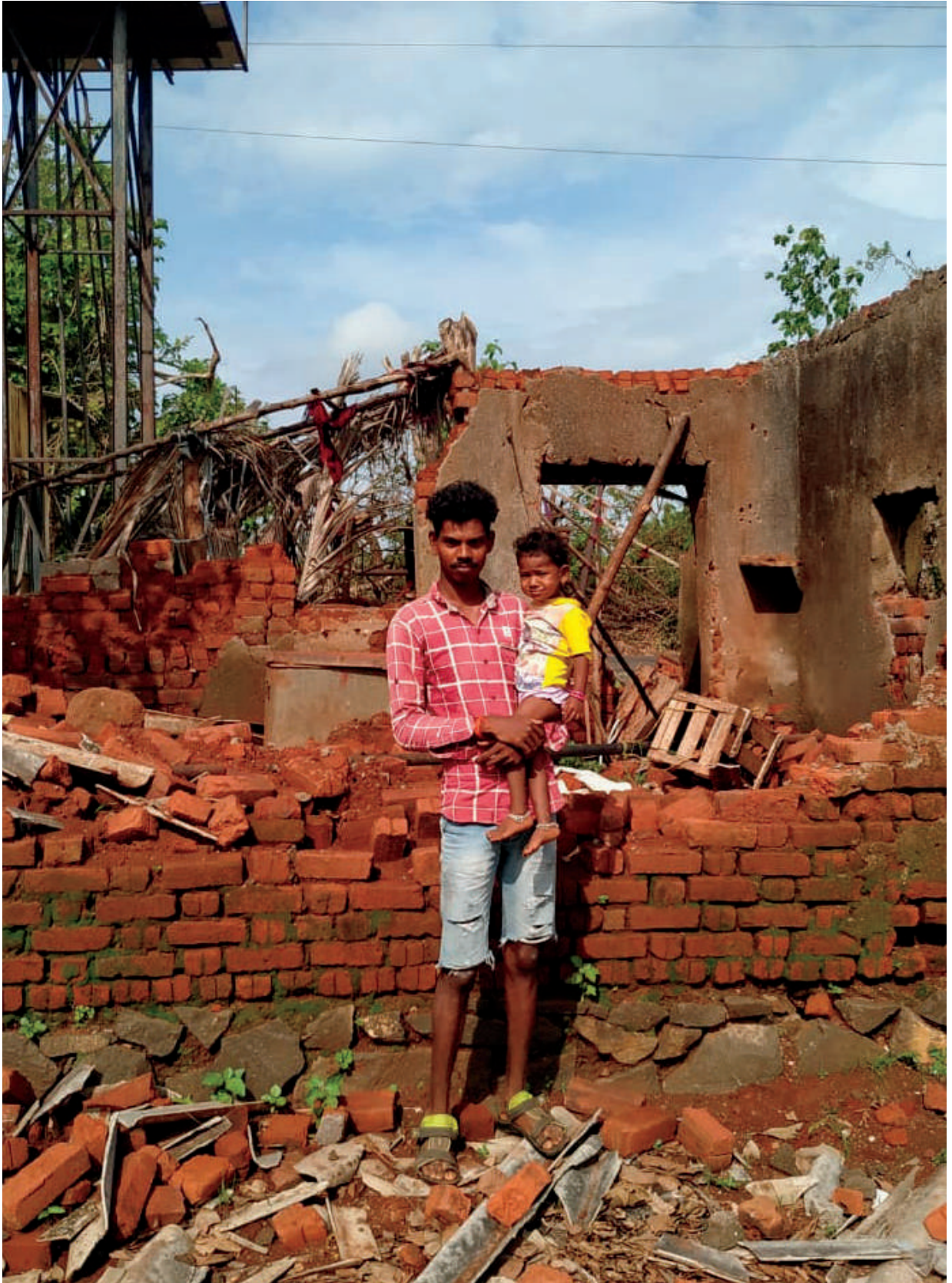
Flooding and heavy rains wreaked havoc on local homes.
