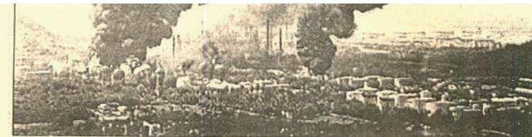
A FULL VIEW OF THE HPCL PLANT ON FIRE/ EXPRESS
