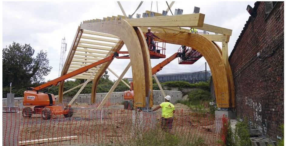
design evolved, affecting the approach to reuse. For example, a decision to reorient the angle of container loading decks, accessed via gaps between adjacent arches, effectively widened the gaps, lengthening the required beam spans and ruling out the use of existing arches over that section of the hall.
