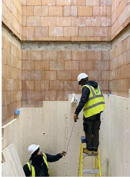
**Left** Poroton blocks form compartment walls. The CLT stair, by Stora Enso, was prefabricated from a kit of parts and then assembled on site.
