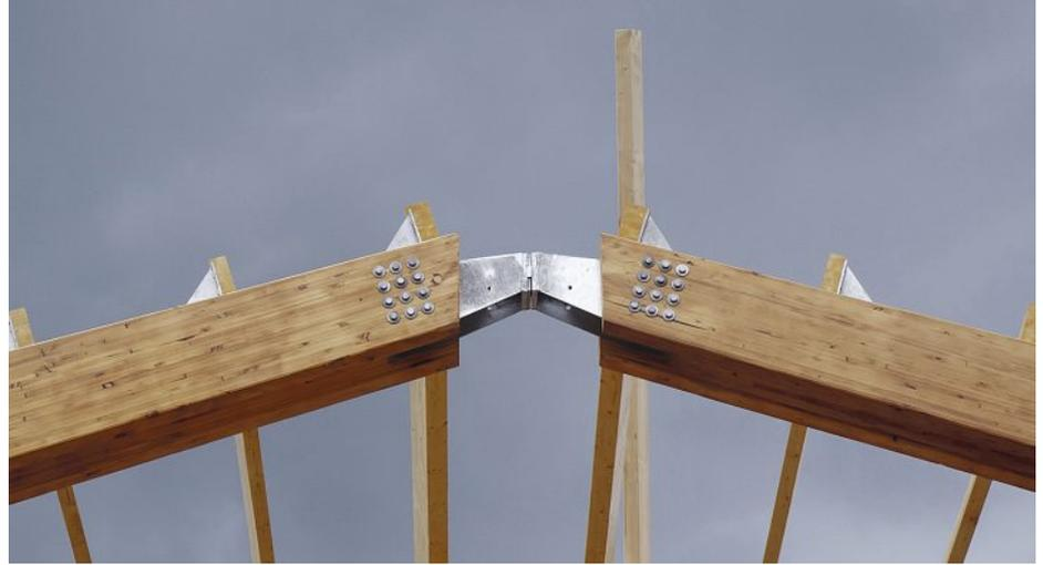
**Above** The tops of the beams were removed, due to rot, and joined with steel connections.
