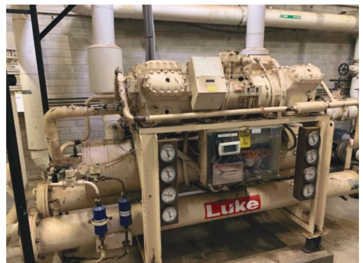
Figure 6 – Original R22 water-cooled chiller
