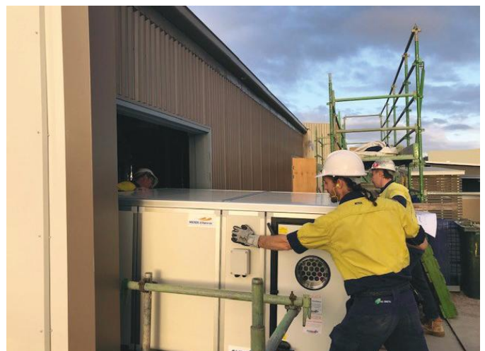
Figure 4: PMU Construction - AHU Installation
