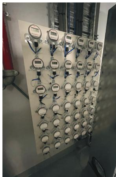
Figure 7: (a)-(c) Various Plantroom Equipment; (d) Differential Pressure Room Sensors; (e) Exhaust Fan Chamber #1
