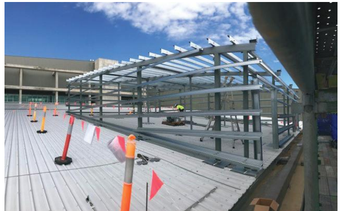
Figure 9: Rooftop Plantroom Construction
