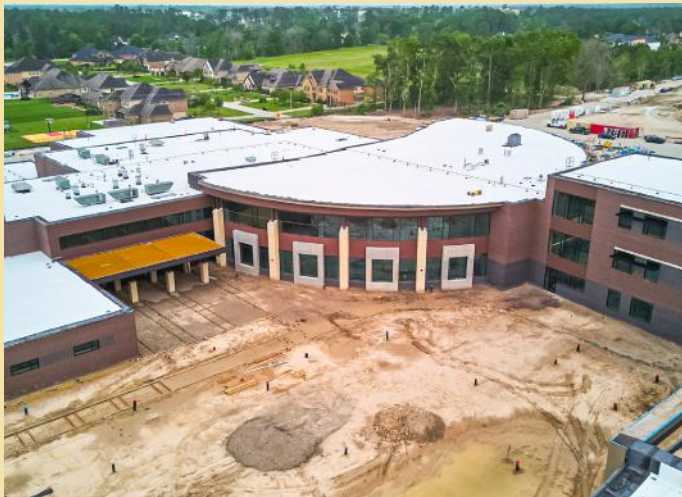
An aerial view of the new Lake Houston Middle School, where over 90,000 sq. ft. of tile and stone were installed using a complete MAPEI system.
