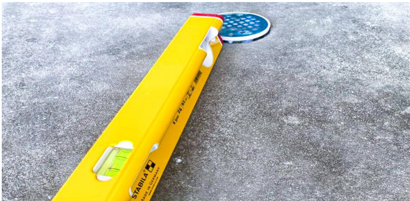
Slope to drain is a core concept covered in the new workshop.
