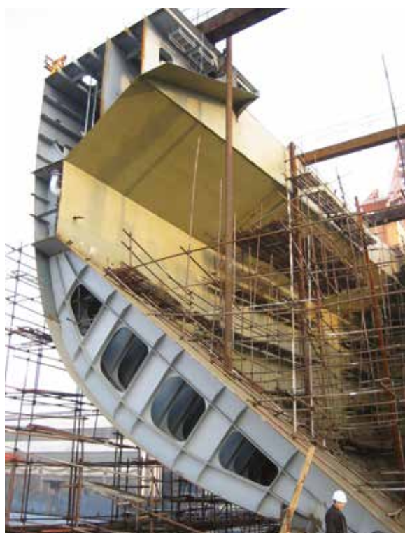
Figure 1.1 Double skin with integral topside and hopper tanks. The after hold of a Diamond 53 vessel
