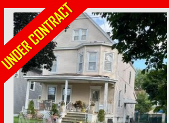
UNDER CONTRACT DE MOTT AVE. CLIFTON
