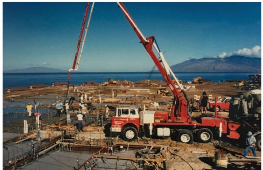
Phase III Building 32 concrete pour. Oct 1986
