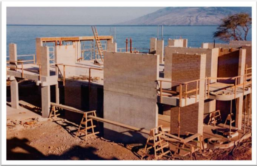
Thick concrete walls of Building 4 form the structural backbone. Sep 1985
