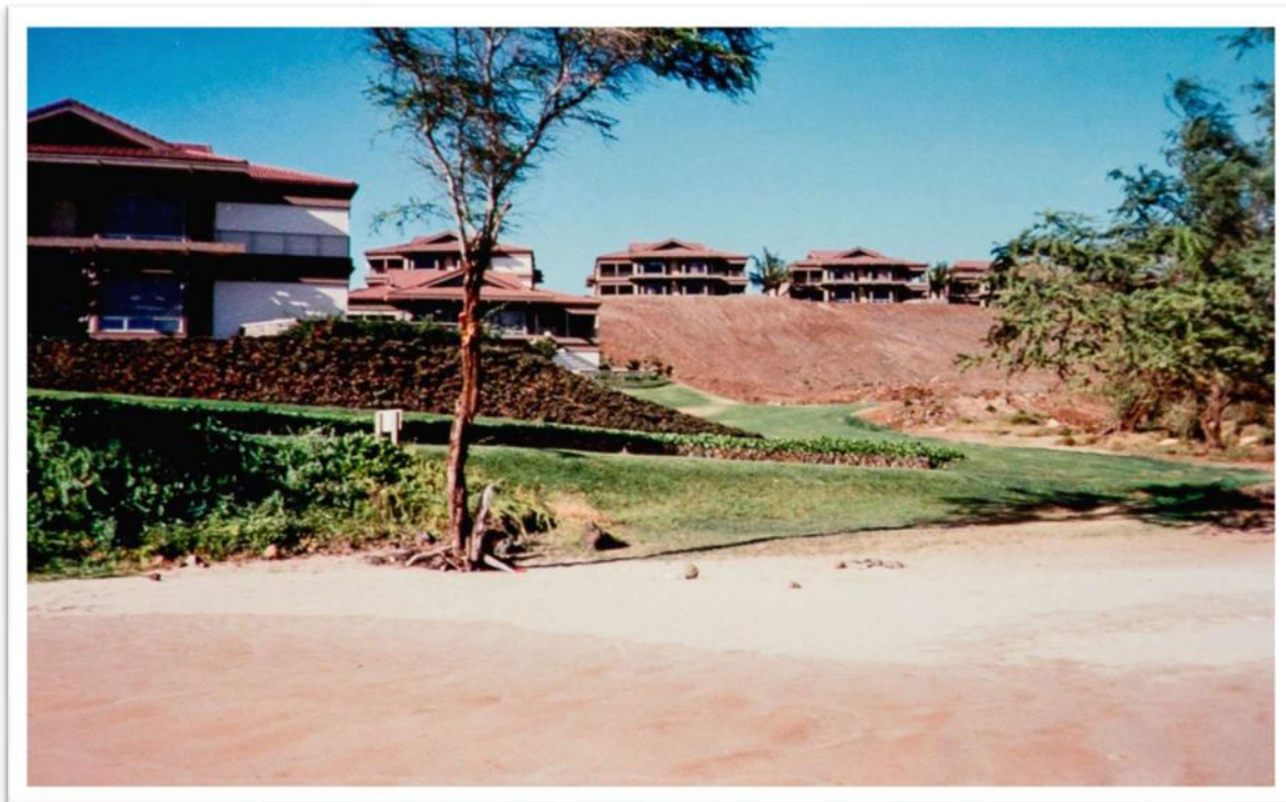
Seen from the north end of Polo Beach are Phase II Building 17, a partial view of Building 18 to its right, and Phase III buildings above that with graded hillside that slopes toward the soon-to-be-built Fairmont Kea Lani. Jun 1987
