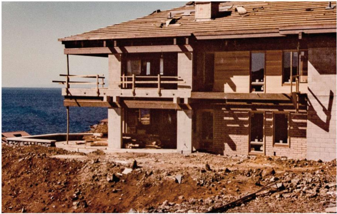
Exterior of Building 32 in Phase III neared completion. Dec 1986
