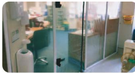
Figure 3. Aluminium frame with industrial plastic walls creating an isolation area.
