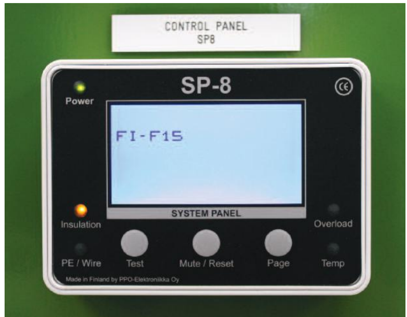
Figure 2. The control panel indicates which socket (F15) the faulty device is in.
