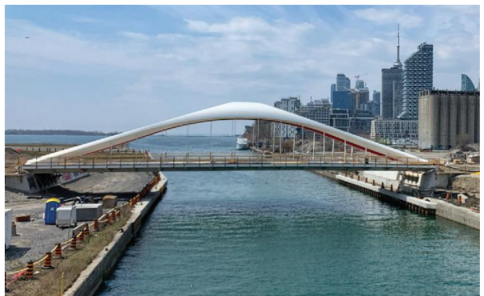
Below: Cherry Street North Bridge in the Port Lands
