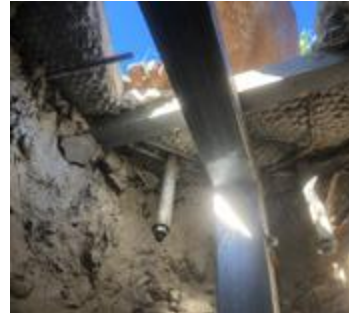
Internal structure of the plinth
