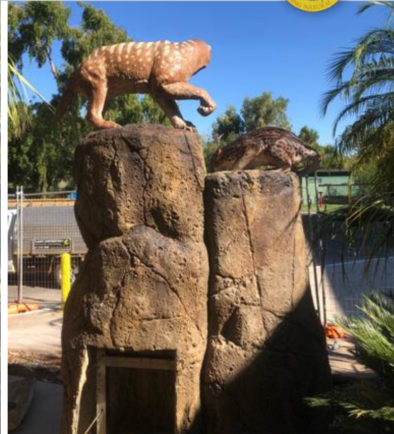
View of rear access door in the rock plinth
