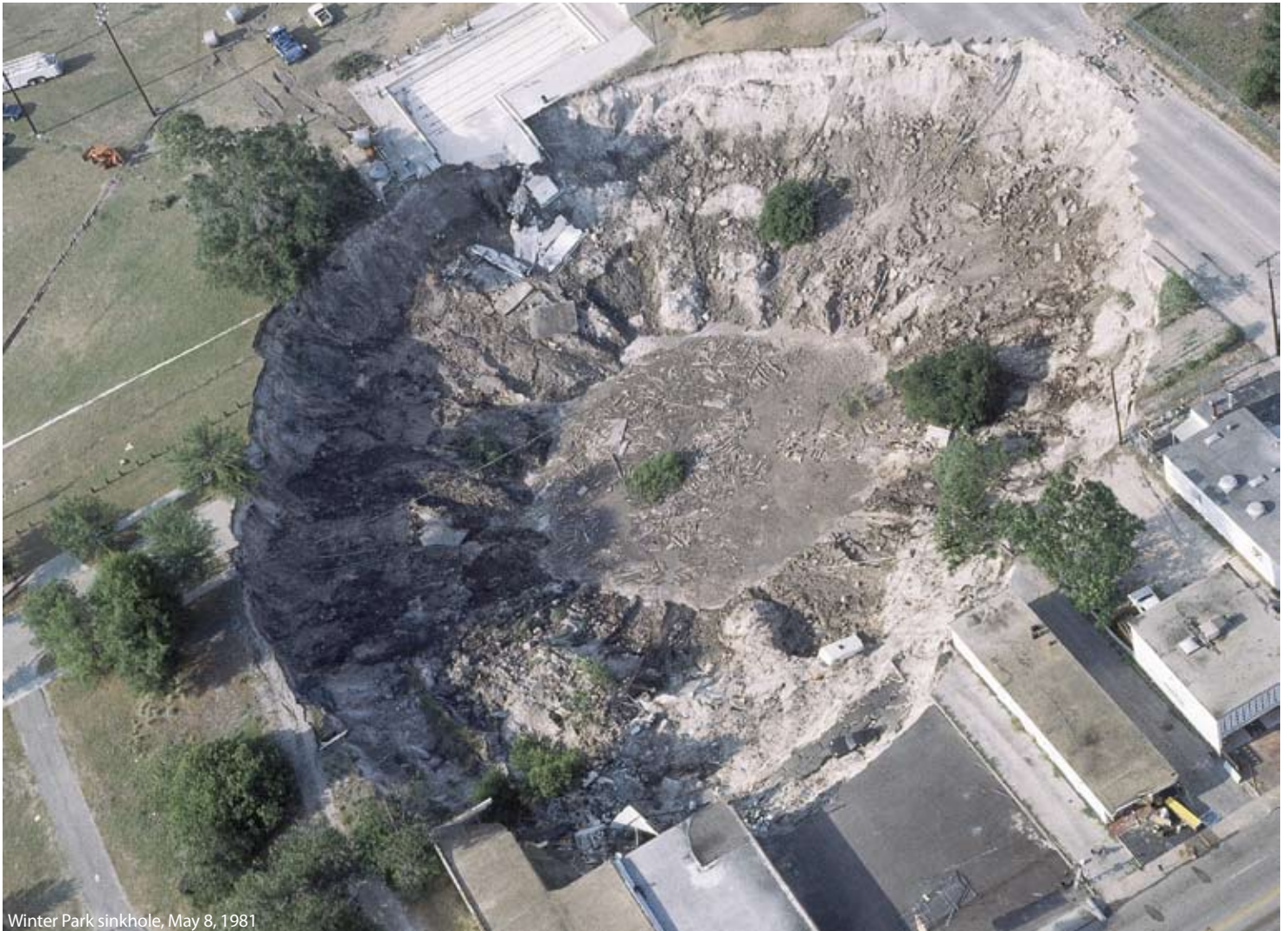
Winter Park sinkhole, May 8, 1981
