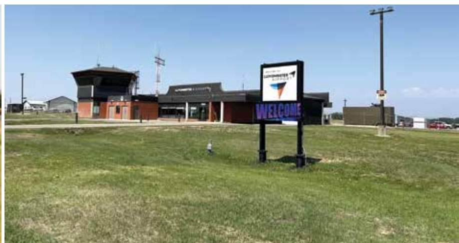
The AAMA envisions a future where these facilities thrive as connectors of remote regions, bolstered by policy alignment and investment. Seen here is the Lloydminster Airport.
