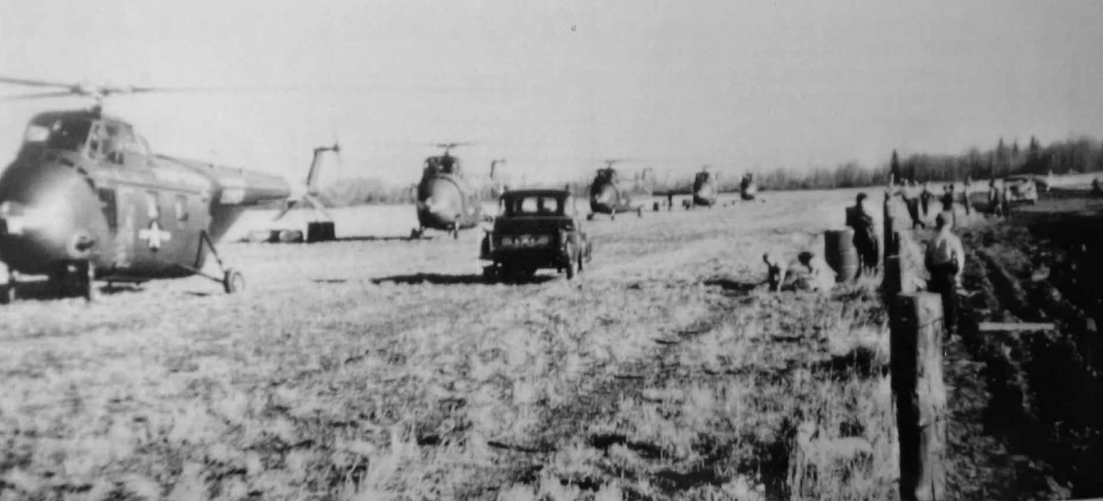
Construction of Distant Early Warning Line in far north brought a flurry of activity to Slave Lake landing strip in 1951-52 when American helicopters made use of it as a fuelling stop.
