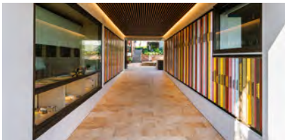
H Block Refurbishment
