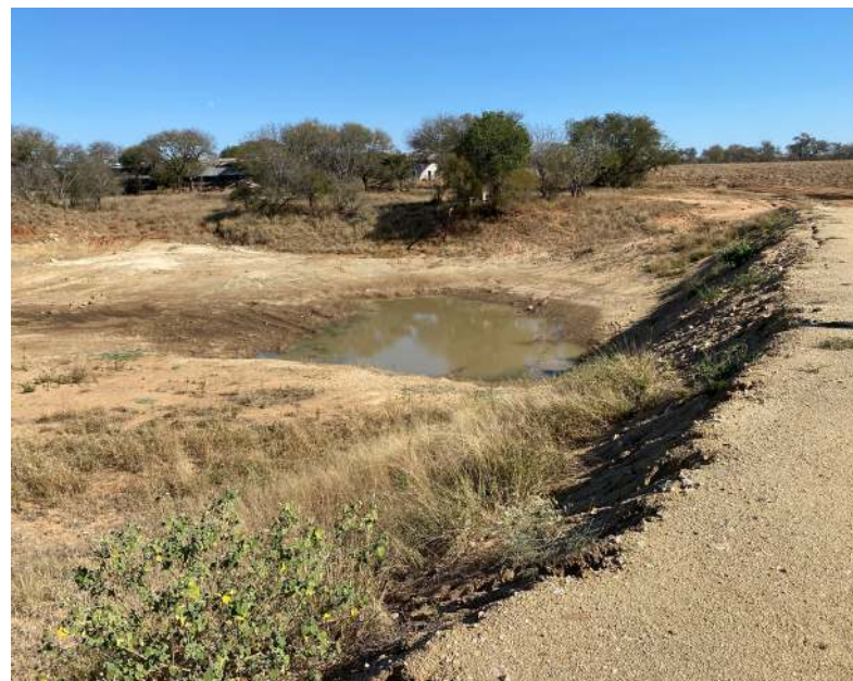
Earthen dam on the farm
