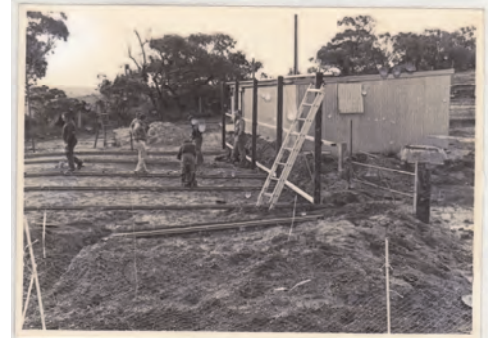
Building the clubrooms in 1979
