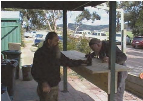
20 July 2011 - Bruce Nettelbeck & Craig Hooper installing Range 6
