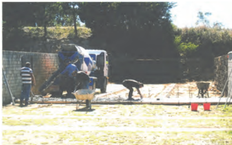
Work on Range 2 upgrades in 2007
