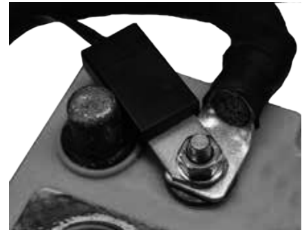
Fig 2.5(b) Temperature Sensor Installation
