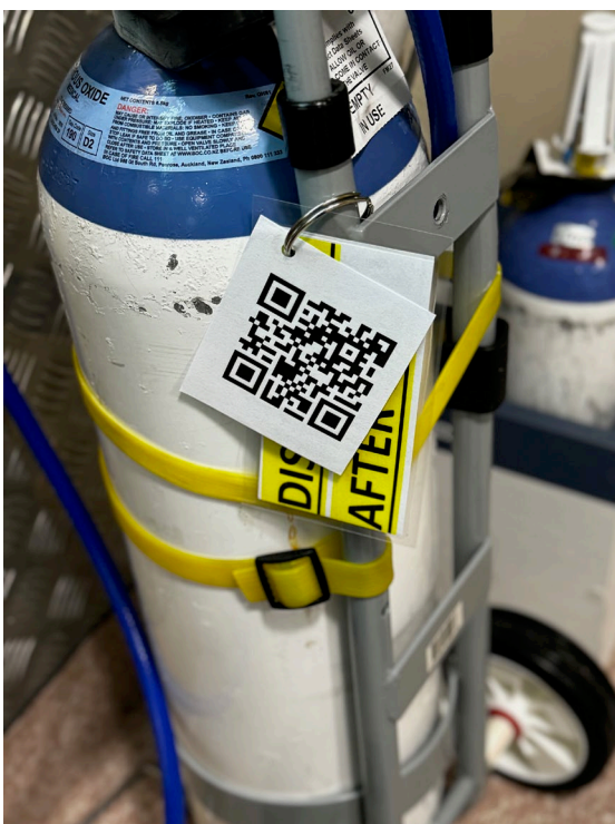
Portable D cylinder with QR code attached for technicians to upload cylinder weight.
