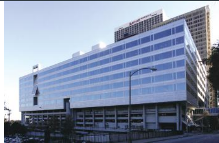
SUNTRUST PLAZA GARDEN OFFICES ATLANTA, GA 30303
