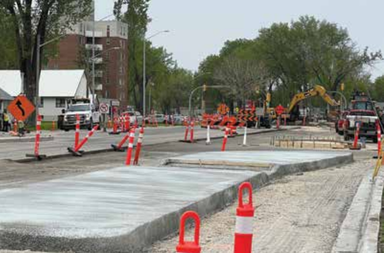
New concrete traffic islands form the protected bike lanes on the north side of Saskatchewan Avenue.
