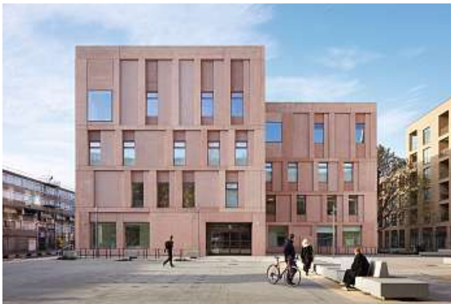
Above: Shifted window openings, varying textures and projecting volumes bring life to what could become a monotonous brief.
