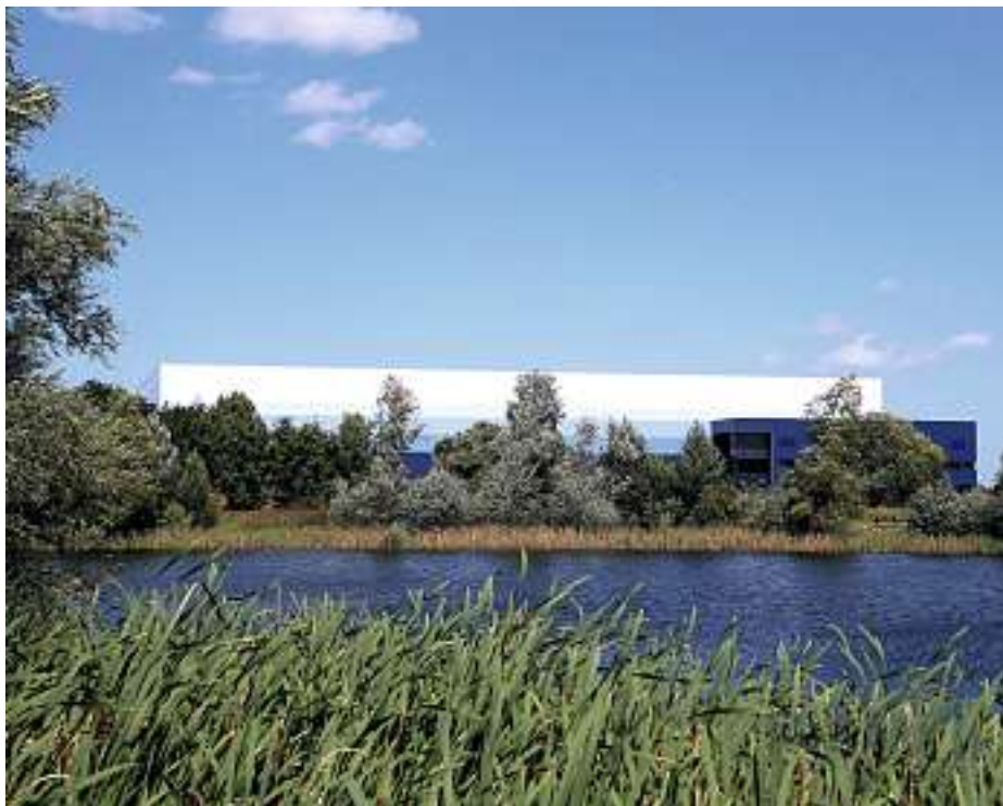
Left: If a shed is not grey then colour may be being used in another way to help it disguise its volume, as at 314 Magnitude Park, Milton Keynes, designed by Chetwoods.
