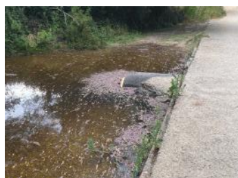
Dolly's Creek Road culvert blockage
