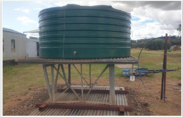
The tank on the stand and anchored down.
