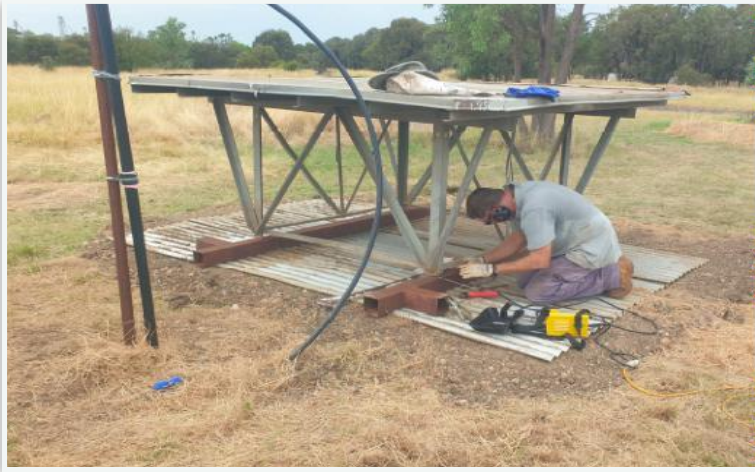
Member Dan welding supports to the tank stand.
