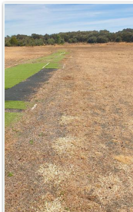
Poor condition of the runway
