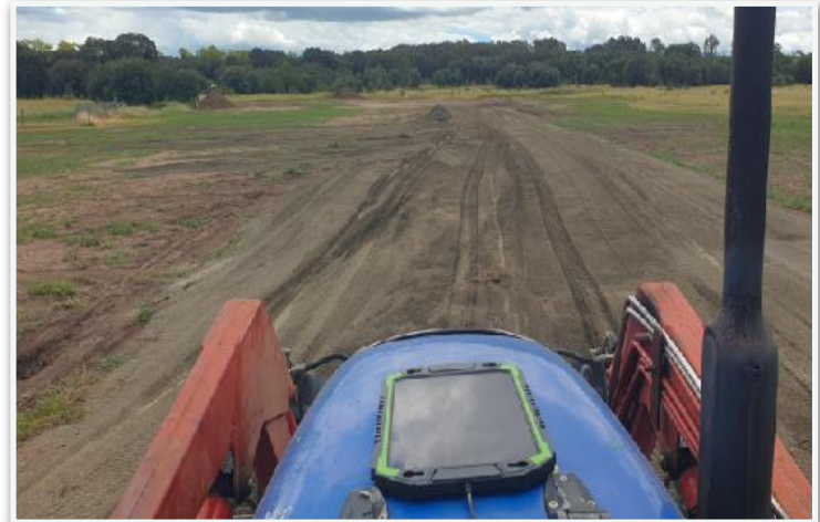
Spreading and levelling of the crusher dust
