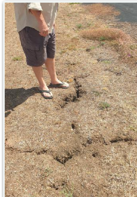
Cracks in the surface
