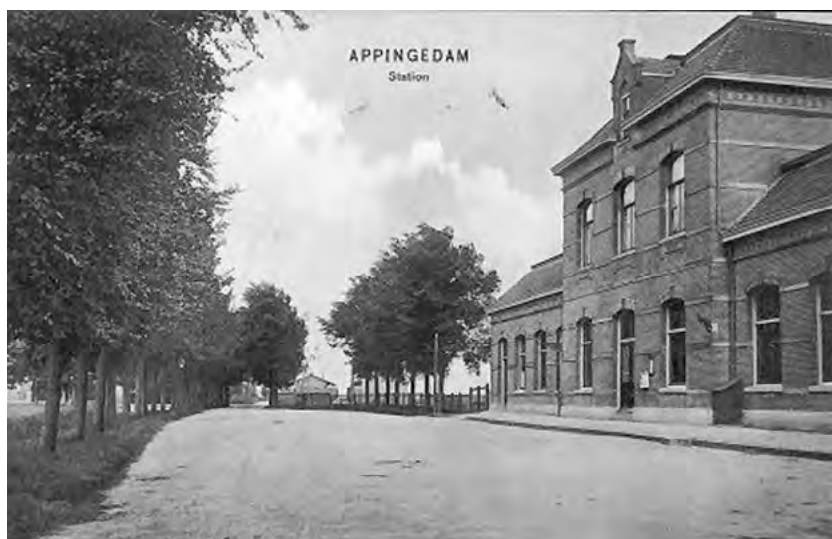
4 Station Appingedam, geopend 15 juni 1884, foto 1900
