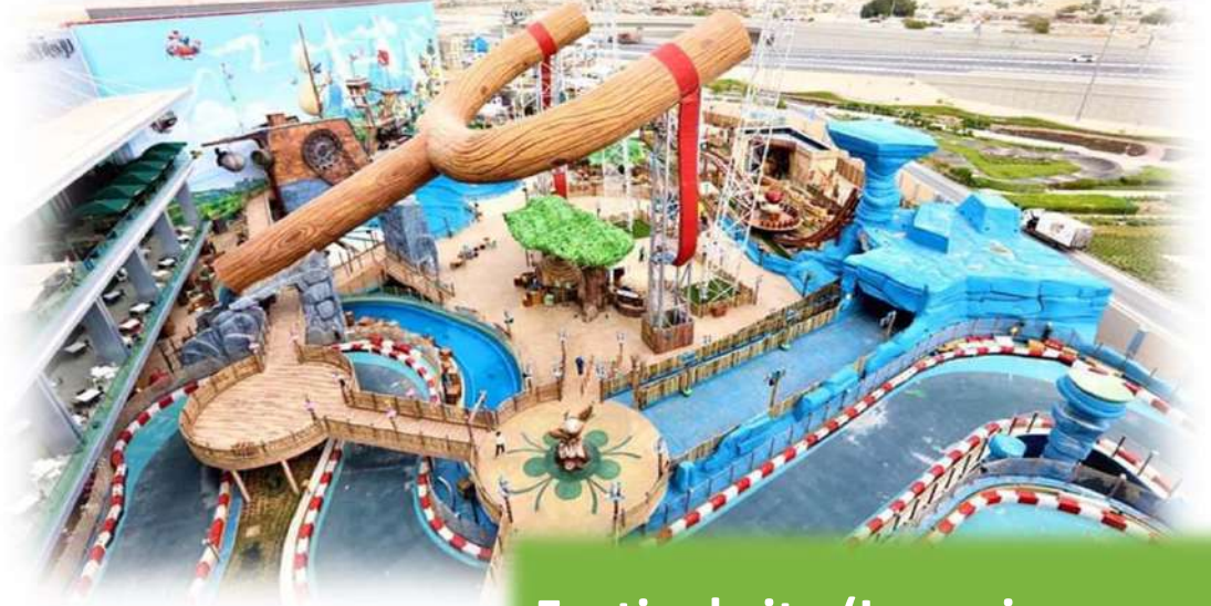
Festival city (Lazy river swimming pool construction)
