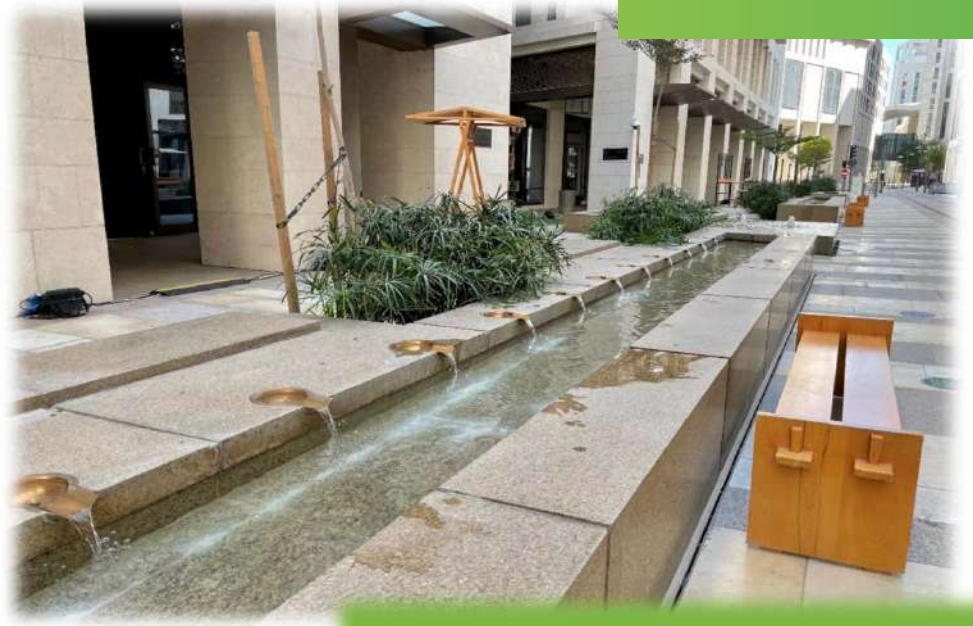
Meshaireb Downtown (swimming pools & Water Features
