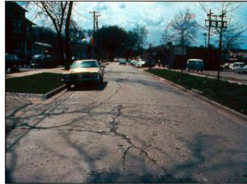
Erratic crack patterns due to no joints
