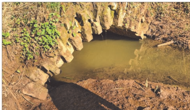
The stonework forming the end of the arch barrel (voussoirs) clearly needs some work by a team of masons
